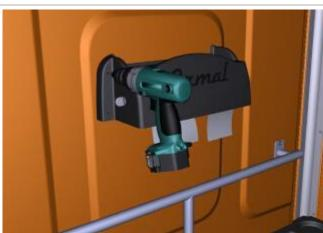
Insert No. 4 rivets from the outside of the restroom to secure the paper holder
